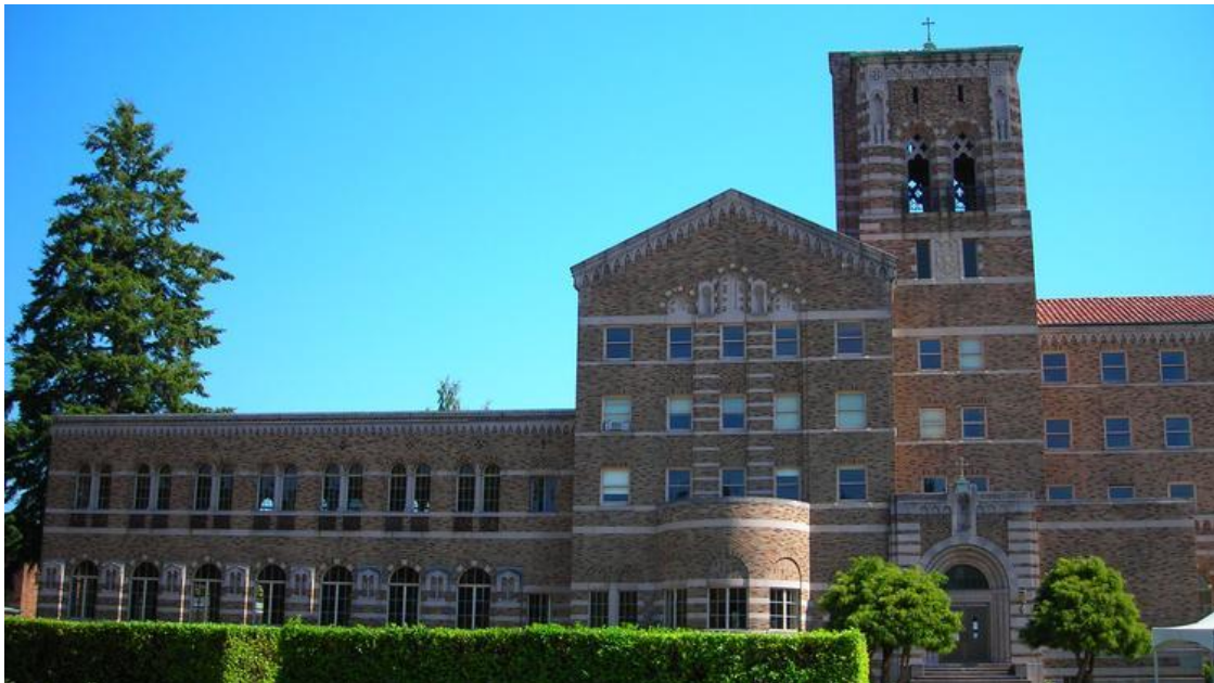
Daniels Real Estate hopes to rehab the St. Edwards Seminary building in Kenmore.
